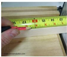
**1g**. Slide the piece, so the mark corresponds with the saw blade.
