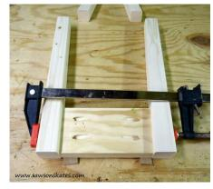
**Step 6.** Attach Long Sides. With the top of the legs facing you, put two pieces of scrap 1/4" material on the workbench in between the legs. Apply glue to each end of a Long Side, place between legs (so the short edge is facing towards you) on top of the scrap, clamp to the legs and attach using 1-1/4" pocket screws. Repeat for the other Long Side.
