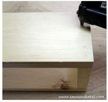
**Step 5.** Attach the Container Front and Back. Apply glue to sides and bottom and attach the front using 1-1/4 finish nails. Repeat for the back.
