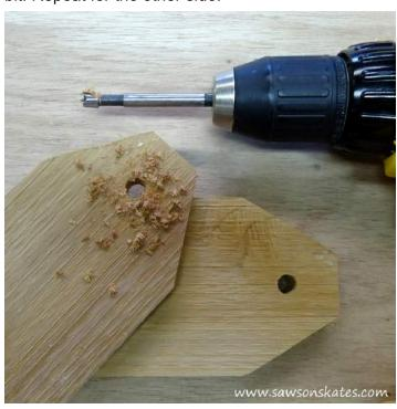
**Step 3.** Cut the Bottom. Cut 1 piece of 1×4 to 12". Drill several holes in the bottom for drainage.
