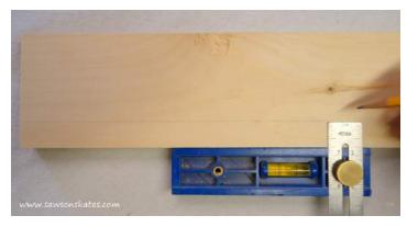
Measure in about 2-1/4" on each side and make a mark. Also make a mark at the middle.
