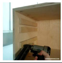
Hold the 13/16" scrap below the support, apply glue to another support, place below the scrap and attach using 1-1/4" brad nails. Remove the scrap. Repeat for the other side.
