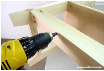
The remaining 3 slats (1x3's from Step 7) are placed so that the tops of the slats are flush with the top of the bottom rails and spaced 13/16" apart. To help with the spacing I cut a few pieces of 3/4" scrap wood and attached pennies to the scrap wood with painter's tape. The thickness of the wood plus the penny equals about 13/16".
