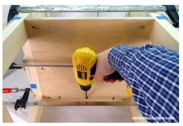
Apply glue to a 1×2 (from Step 6), place at the top of the back legs and attach using 1-1/4" pocket screws.
